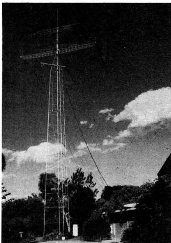
The VK3BM antenna farm—a TH6DX beam at 100ft and a home-built full-size 7MHz Yagi at 86ft supported by a lattice boom being the main features
